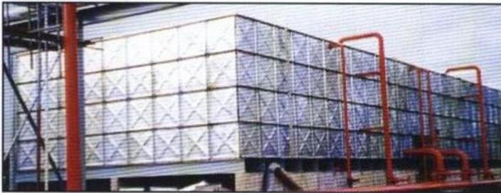
Tank on dwarf walls with steel skid beam
