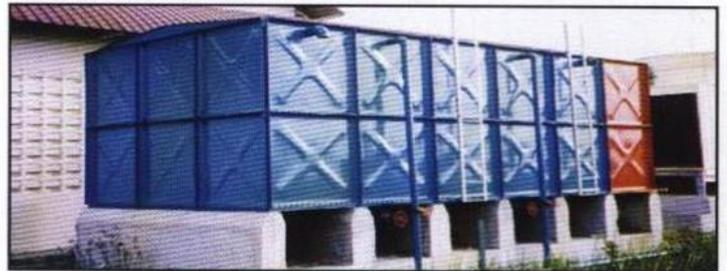
Tank on dwarf walls without steel skid beam
