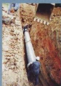
Pipe laying in East Malaysia
