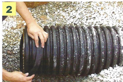
2 Insert rubber ring onto second valley of the pipe
