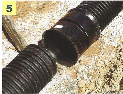
5 Align the next pipe with the socket and repeat Step 1 and 2
