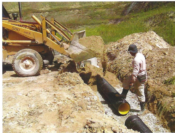
Backfilling of sewer pipe
