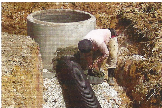
Grouting WEIDA DWCP to a concrete manhole
