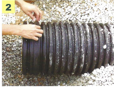
2 Insert rubber ring onto the second valley of the pipe
