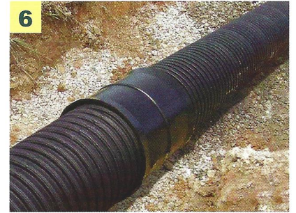
6 Pipe is pushed into the socket to complete the connection
