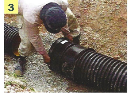
3 Align and insert socket into pipe
