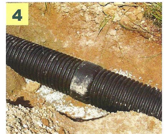
4 Example of a complete connection
