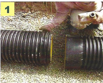
1 Clean pipe end, rubber ring and internal faces of bell end with soap water
