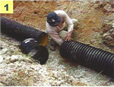
1 Clean pipe ends, rubber rings and internal faces of the socket with soap water
