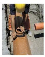
3 Screw the ring nut with the appropriate clip until the blocking of the obtained branch.
