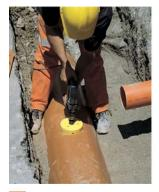
Drill the pipe squarely with a cylindrical saw ø = 152mm (6").
