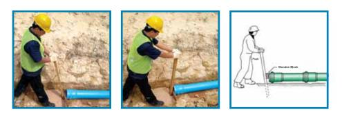
While keeping the lengths in proper alignment, brace the socket and push the spigot into the bell. The spigot should be inserted until the reference mark on the pipe barrel is even with the edge of the socket.
