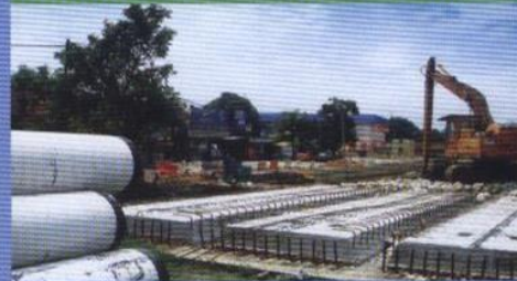
PIPE RELOCATION AT ROAD UPGRADING PROJECT
