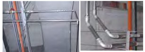
Internal Plumbing (Pipes install at ceiling)
