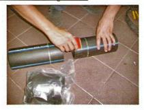
Clean up the connection part. Marked the inserting depth on the pipe end. Scraped and polished the jointing surface. After polished, prevent the jointing surface from contaminating especially touching grease and dirt.
