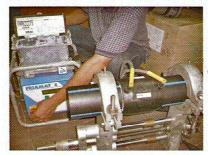
3. Connect the control units leads to the terminals on the fittings. Switch on the control unit. Some automatic units will have sensor which can acknowledge the coupler and do the welding automatically. If not, manual machine will have to be done by turning a few button. Please refers to the control unit supplier for proper guide on this step.
