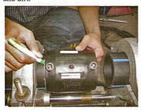
Insert the electrofusion into both pipe ends.
